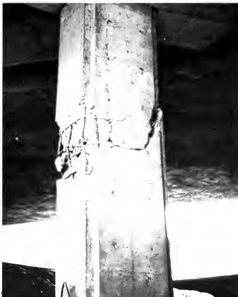
Photo 5. Shear failure in column of San Fernando Road overhead [2].
